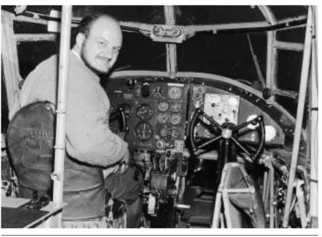
Malcolm Payne in Anson DA. The undercarriage crank handle is to the right of the throttle levers, and the two green gear indicators are just forward, peeping from under their flaps.
